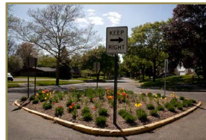
Use of greenery along major routes helps collect storm water runoff and create a sense of place
