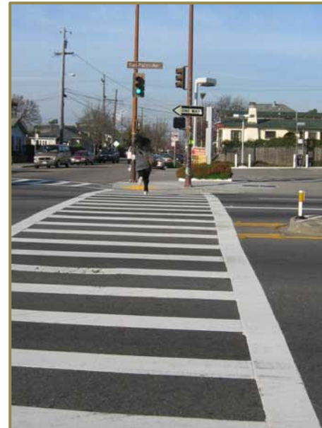
An example of a painted intersection, safe for pedestrians
