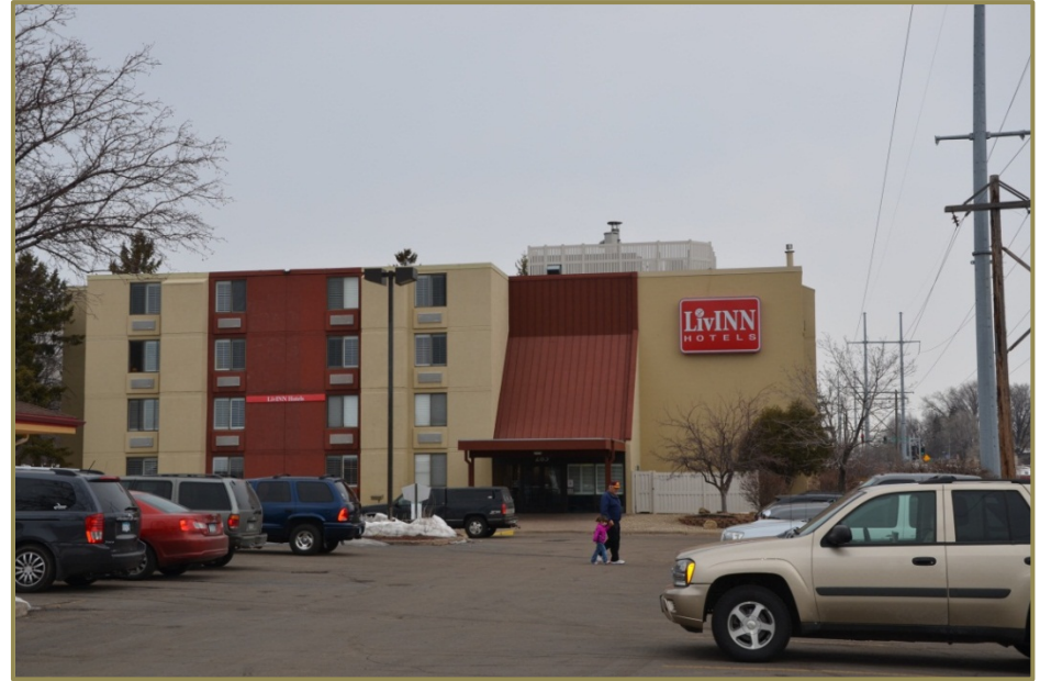
Current hotel site along Tanner's Lake with parking directly abutting the lake
