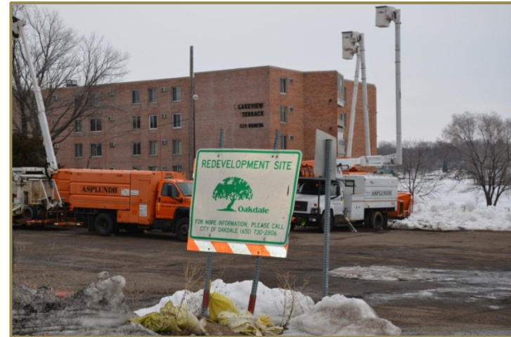
Oakdale's sign along the West Bank of Tanner's Lake designating the area as a redevelopment site
